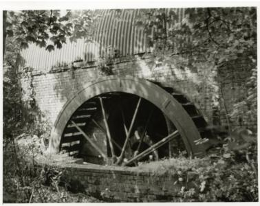
WAI 159-5 1972 The exposed water wheel with most paddles intact
