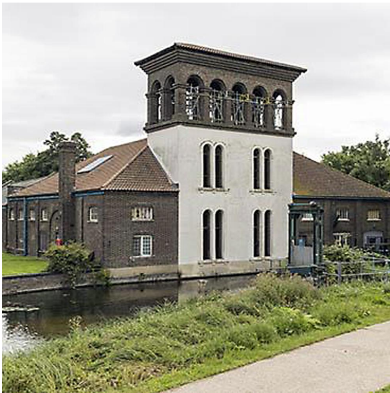
Marine Engine House and Swift Tower
