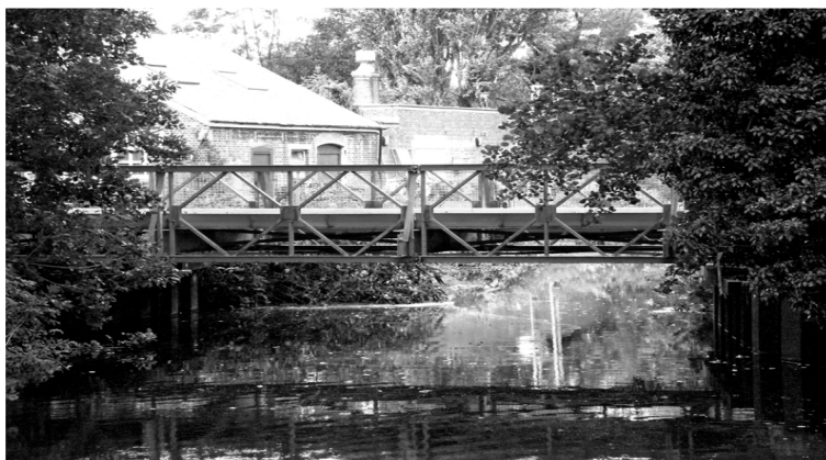
Bailey Bridge next to Powerhouse
