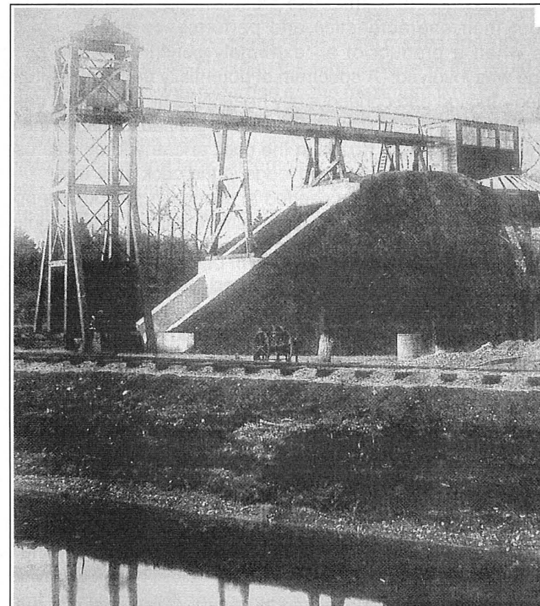
E2 Nitrating House No.1 (circa 1900) showing Acid/Glycerine lift with 'Tramway' in foreground
