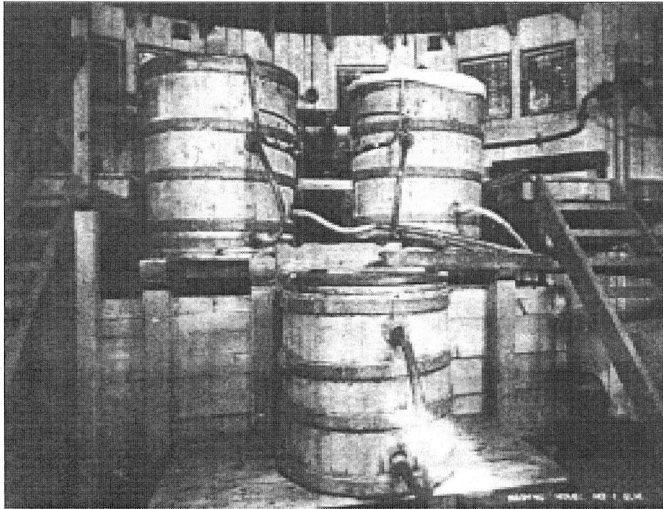
1903 Quinton Hill Nitroglycerine Washing House Washing tanks on upper platform and Filtration tank on lower with a Drowning tank below the Washing tank.
