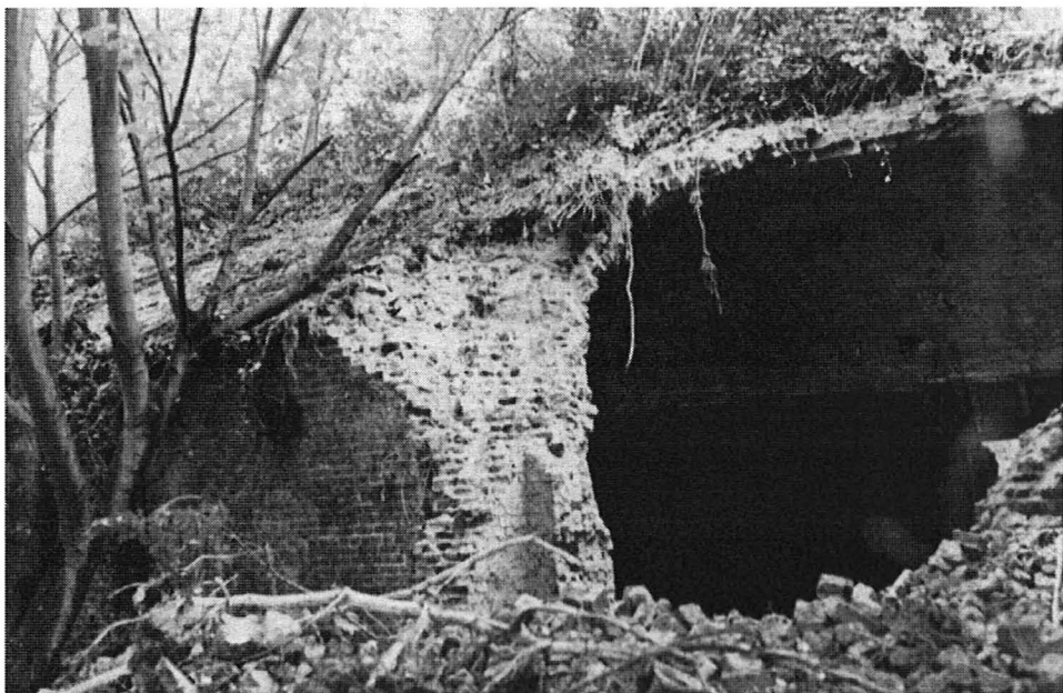
The central main storage area showing results of illegal brick removal
