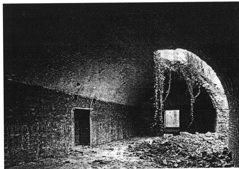
Interior of the central main storage area showing results of illegal brick removal The MoD Police caught a builder who had broken in at the North end of the Site and was in the process of demolishing the building for the bricks!
