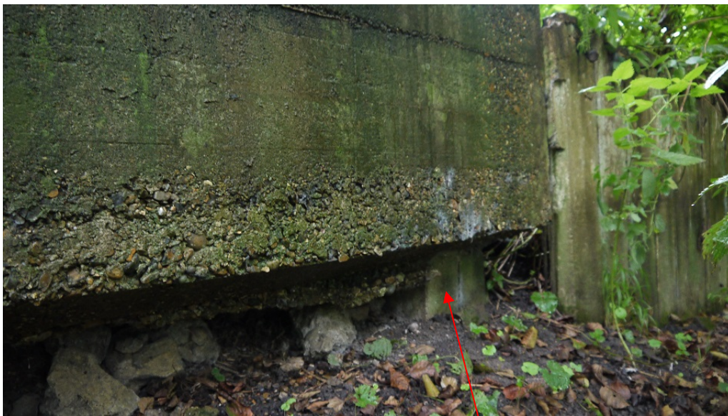
7. Top of concrete pile exposed by ground erosion
