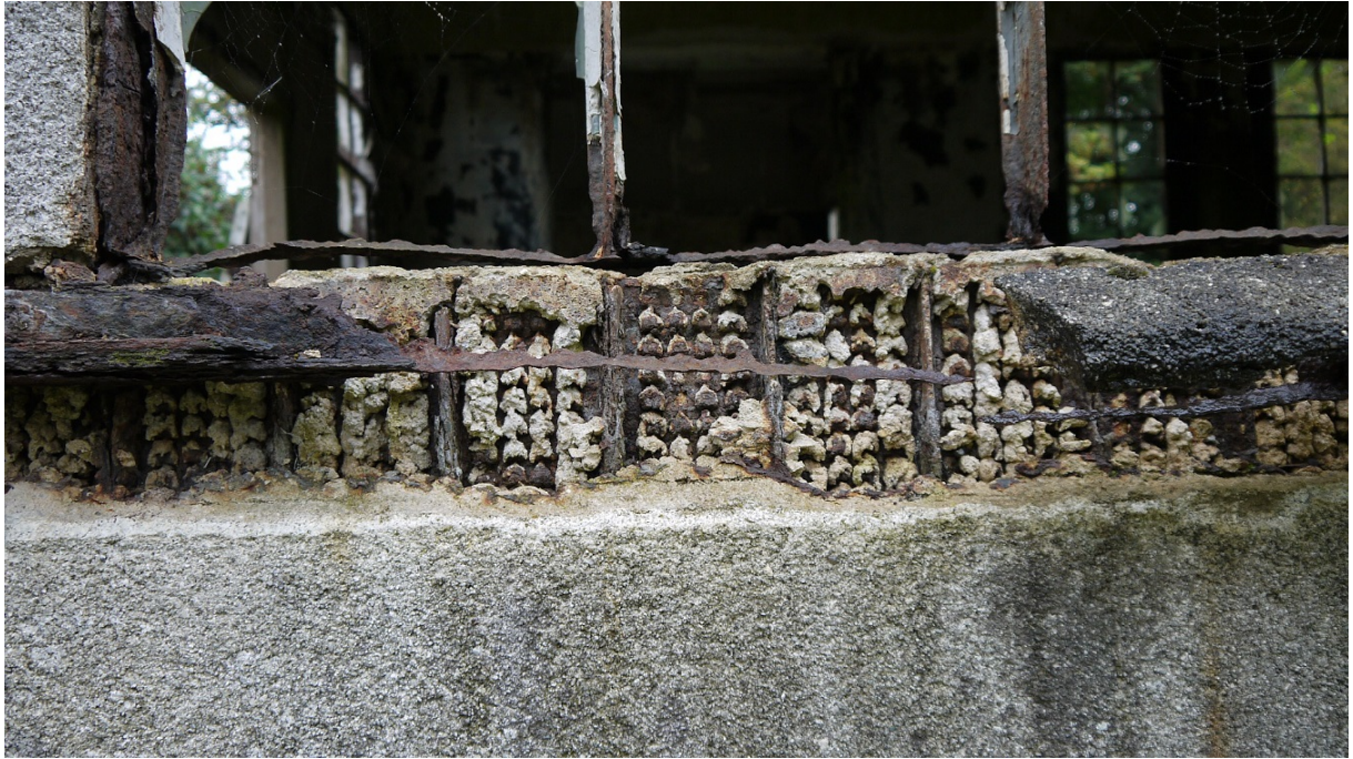
2. Detail of the ribbed lath wall at window cill level. The horizontal angle has completely corroded
