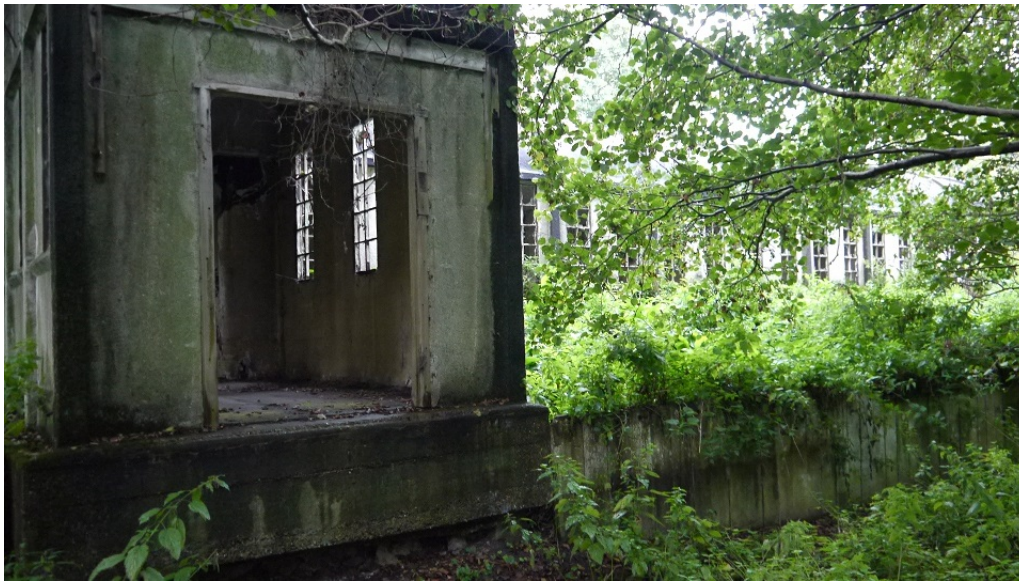
6. Edge of slab undermined by ground erosion
