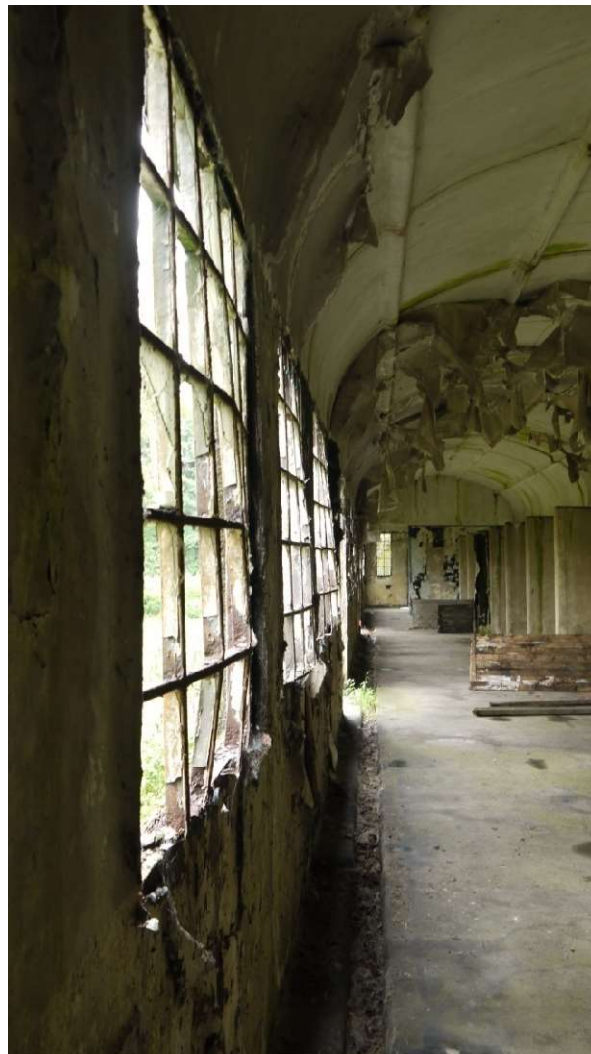
4. Inside of east elevation showing bow in wall
