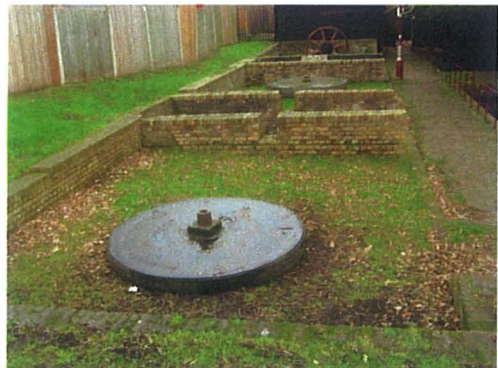
Two other stone beds for a pair of mill wheels are illustrated here.
