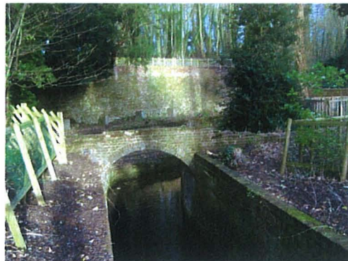
Brick / stone lined canal
