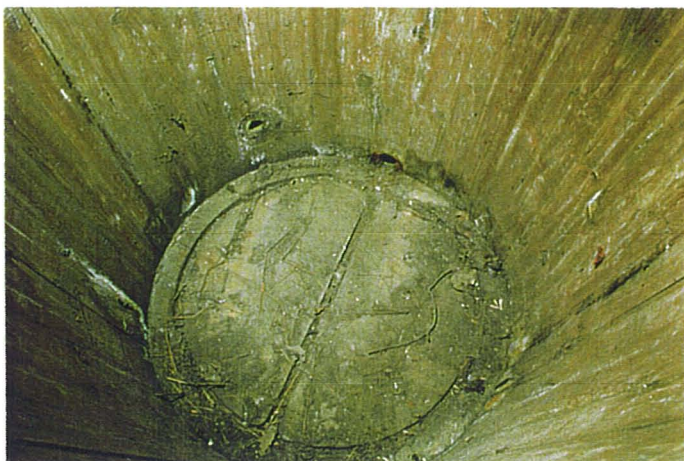
Plate 27 Interior detail of a washing tank, showing nitroglycerine and wash water drainage outlets and grooves in the base of the tank. The lead lining has been removed
