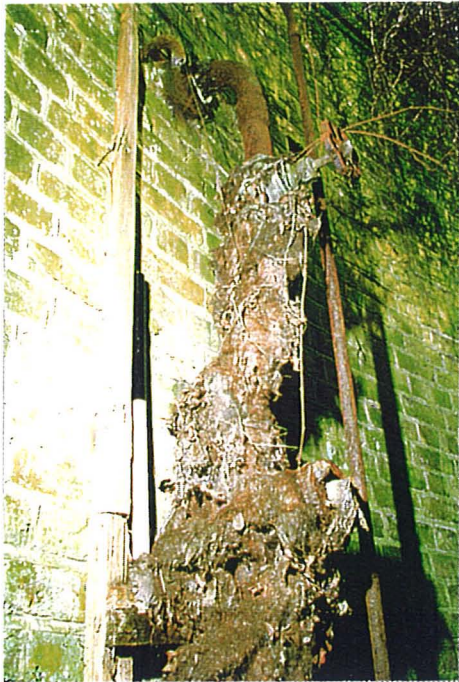
Plate 15 Asbestos covered pipe and stop cock, probably connected to the Washing House steam heating system
