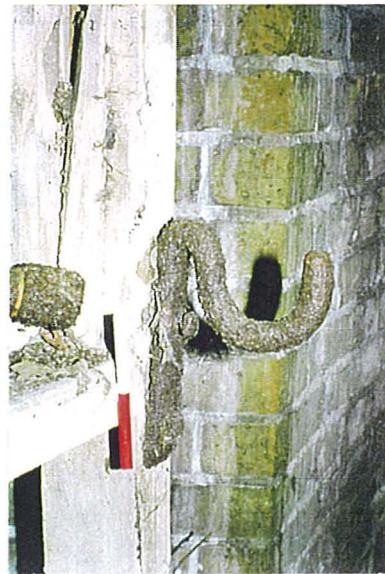
Plate 37 Detail of an iron hook attached to the wall of the southern conduit tunnel. It is one of a row of identical hooks running along the E side of the tunnel, probably intended to carry a water pipe.
