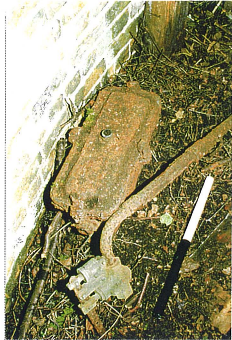
Plate 16 Radiator heater unit, no longer connected, but close to its original position
