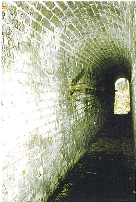
Plate 36 View along the southern conduit tunnel (looking S). The row of iron brackets set into the E wall formerly supported the nitroglycerine gutter
