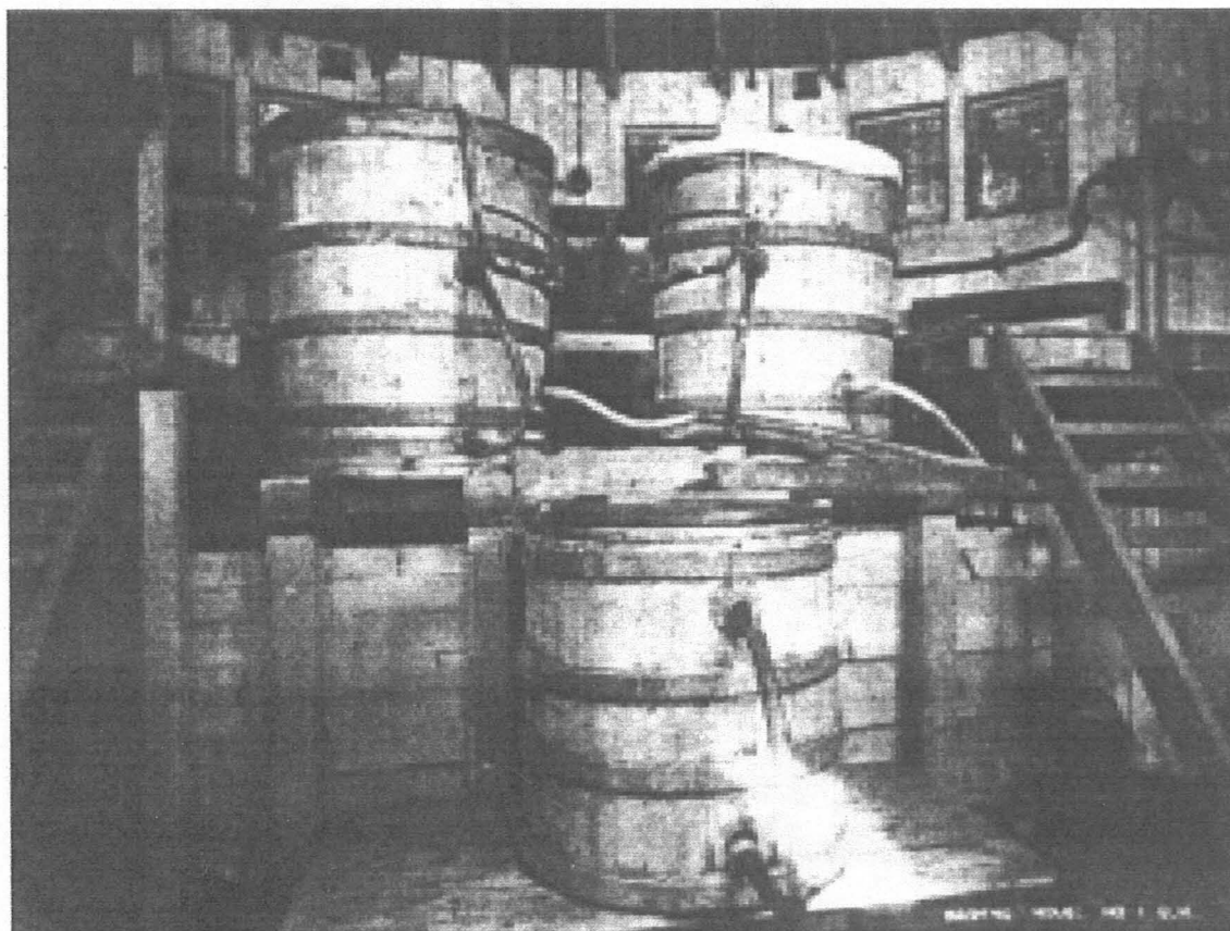
1903 Quinton Hill Nitroglycerine Washing House Washing tanks on upper platform and Filtration tank on lower with a Drowning tank below the Washing tank.
