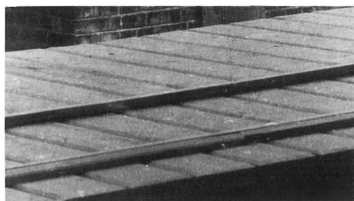
Metal-clad wooden rails; a detail from a photograph taken in 1892 at the Group G gunpowder mills. (RARDE)
