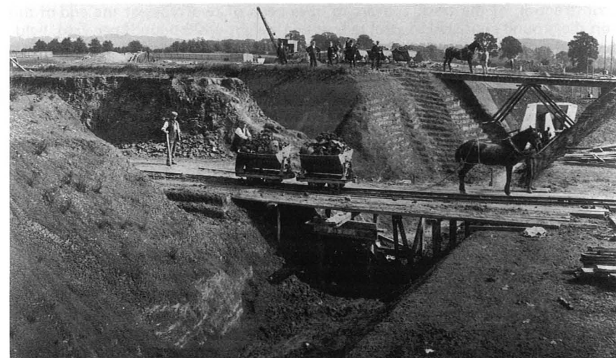
Horse-drawn tip wagons in use during the construction of the South Site cordite stove complex in the 1890's. (RARDE)
