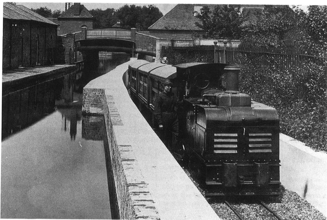
A photograph taken in 1917 showing a train travelling south, with the road tunnel in the background. The railway was 3ft below the river level where it passed under Highbridge Street, and the substantial wall separating the railway and river is apparent. The locomotive is one of the 1917 Ruston Proctor petrol-paraffin tractors. When this photograph appeared in a Ruston Hornsby publicity hand-book, the gauge of the railway was wrongly given as 2ft. (RARDE)
