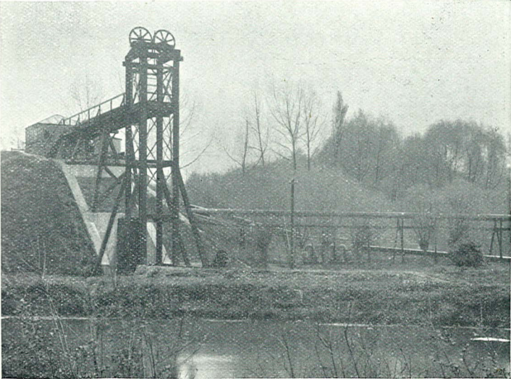
A NITRO-GLYCERINE LIFT. Showing Earth Banks round N.G. House.
