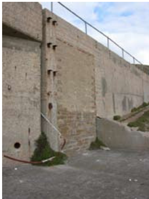
Figure 20 Gantry 1 showing the blocked High Test Peroxide bay and the vertical joint separating the gantry foundations from the causeway. (c) English Heritage
