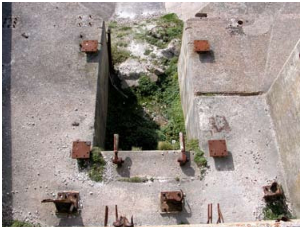
Figure 19 Gantry 2 detail showing the fixing plate for the gantry and efflux duct beneath. (c) English Heritage
